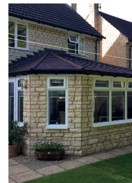
Timber Tiled Roof
