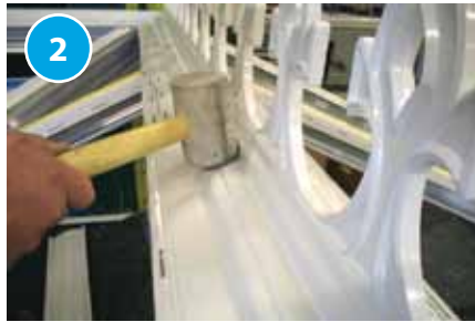
2 Starting at one end knock the top cap in to position using a rubber mallet.
