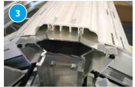
3 The top cap is in it's correct position when the wings of the top cap touch the wings of the main ridge.
